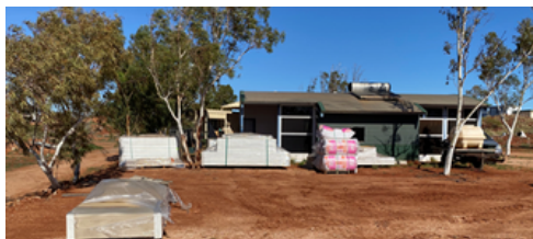
Stage one material onsite
