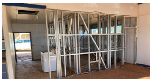
Demolition internal walls
